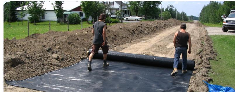
The SX Series includes several woven geotextiles with different manufacturing processes. These geotextiles are specially designed to perform the function of reinforcement, filtration, or a combination of reinforcement and filtration, under structures with high mechanical loads. Due to their specific manufacturing process, woven geotextiles have high mechanical strength, low elongation and filtration capacity to limit the development of rutting in reinforcement and filtration applications.
