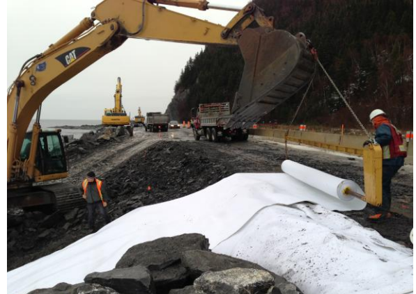
Figure 4 – Geotextile installation on a slope using an unwinder
