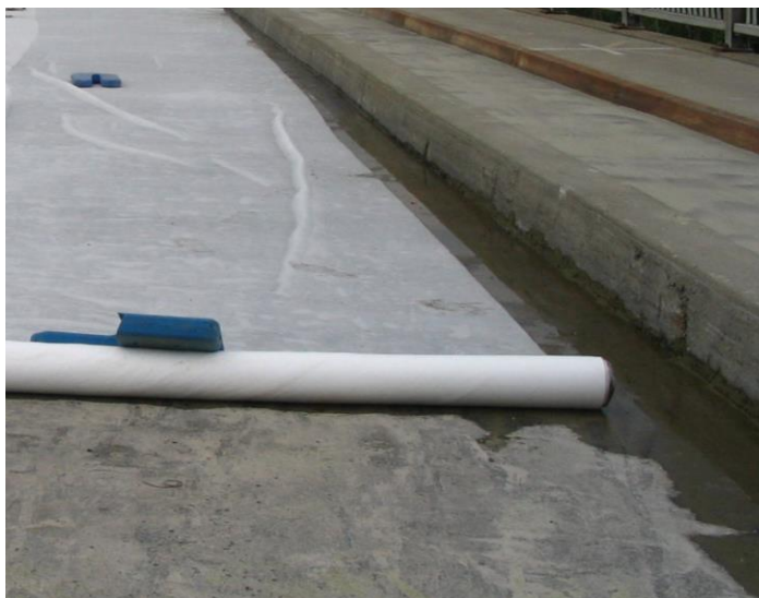
Figure 1 - Installation du TEX-CURE
