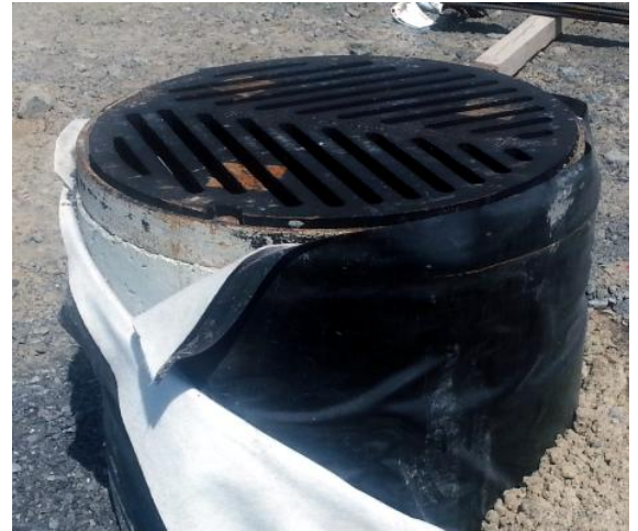
Figure 1 – Tex-O-Flex with the PVC geomembrane facing outward
