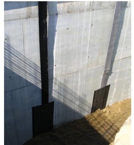
Figure 7 – Installing TEXDRAIN 80H for bridge abutment drainage
