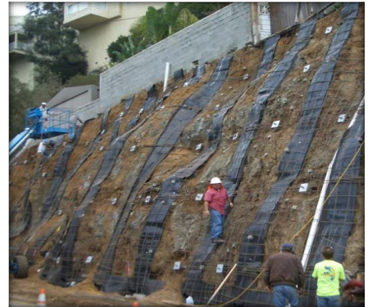
Figure 8 – Installing TEXDRAIN 80H as a drainage shield on a rock face
