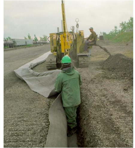
Figure 5 – Laying TEXDRAIN 80V with a trenching machine
