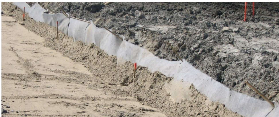
Figure 2 – Installation of TEXDRAIN 80 V for road use
