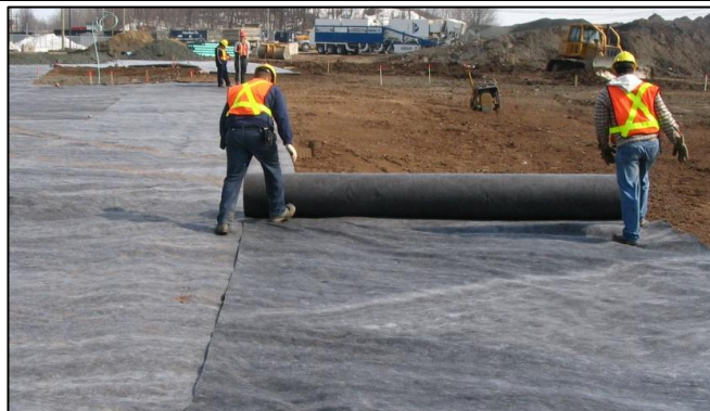
Figure 1 – Installation of Texel Géo-9
