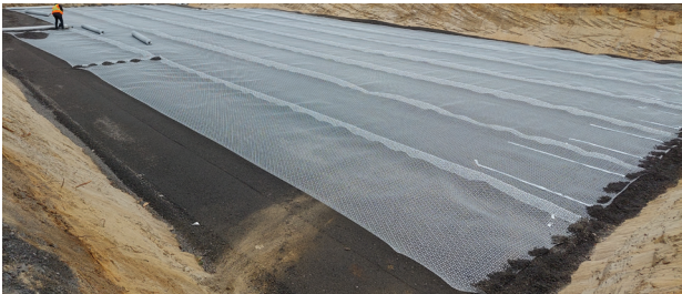
Installation of NXST Geogrids
