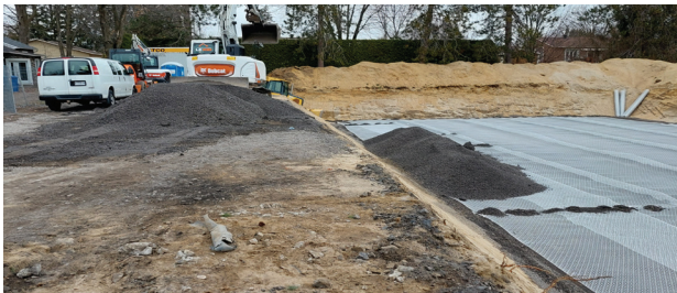
Placement of Fill Material Over the NXST Geogrid
