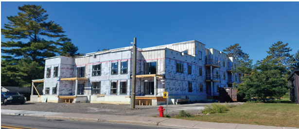
Building Under Construction
